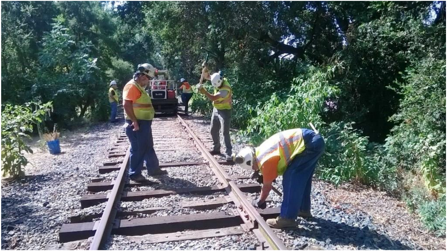
Clem sets spikes as Kyle drives 'em home
