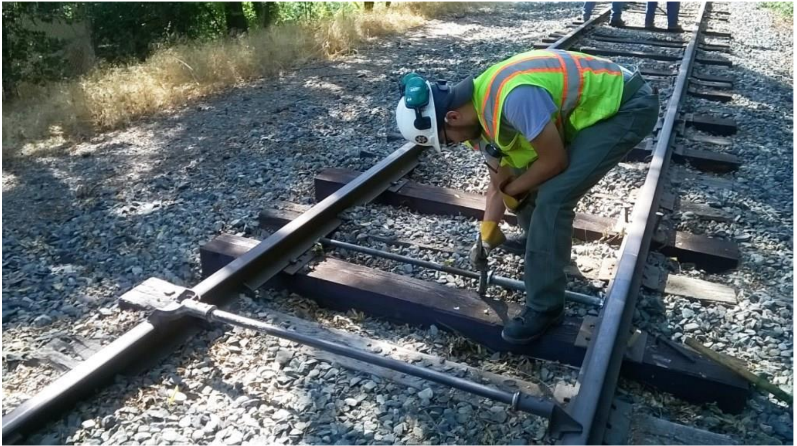
Using the rail-spreader, Kyle brings the rails back into gauge
