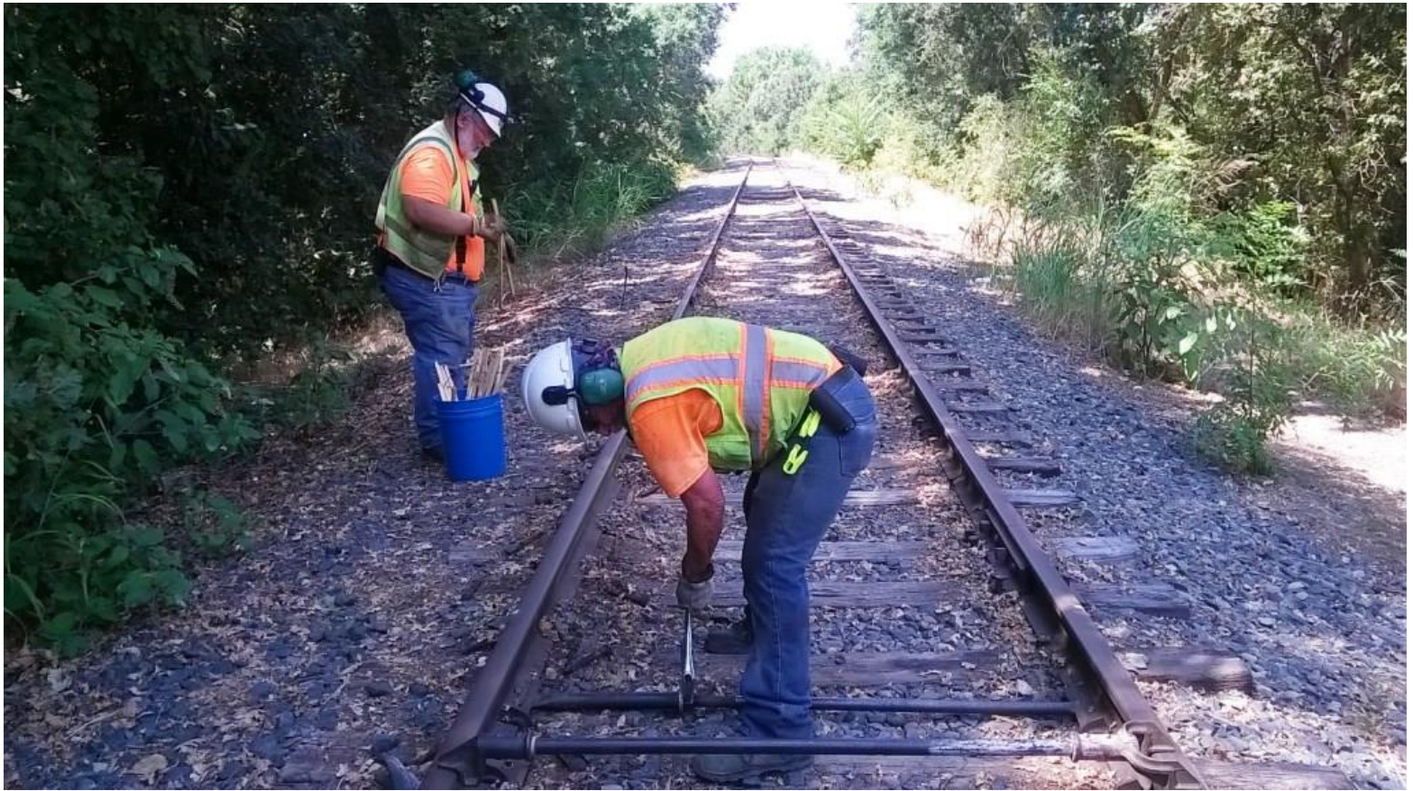
Frank plugs spike-holes in ties as Joe uses the rail-spreader to bring the track into gauge
