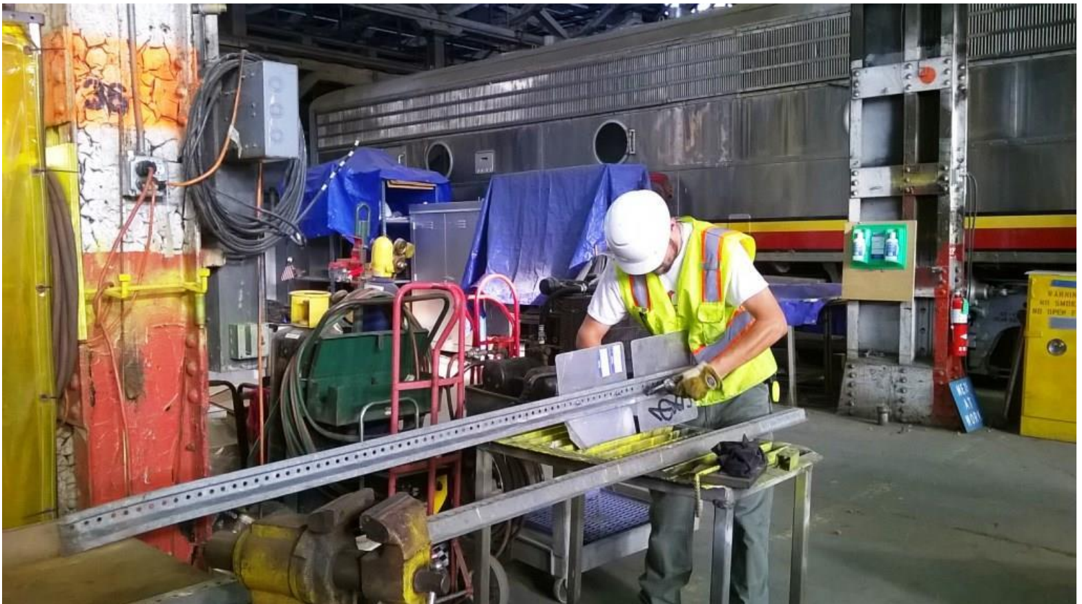
Kyle works on repairing the whistle boards
