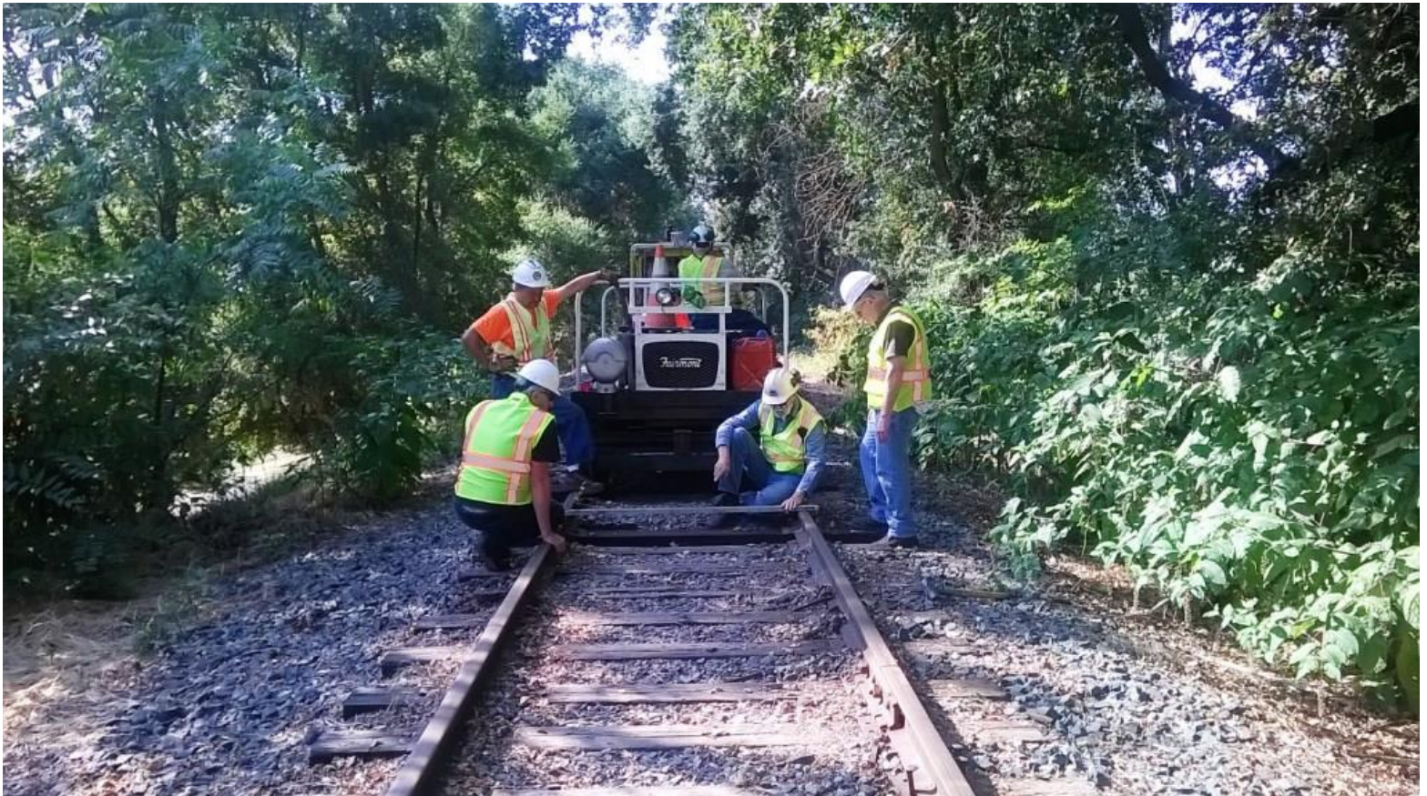
Alan demonstrates for Bill and Scott how track is re-gauged
