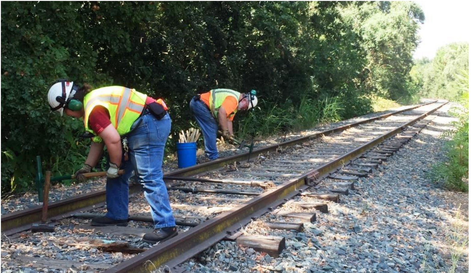
Heather and Frank drive spikes at the re-gauged rail
