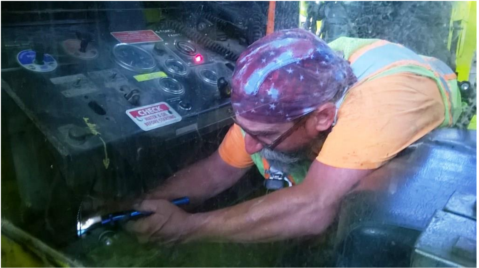
Joe fixes the man-lift's incessant electrical problem
